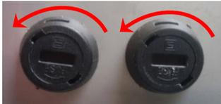
*Figure 22: Replacement of the fuses*
